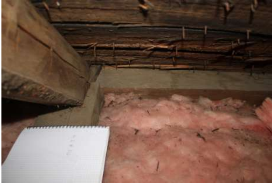
Photo 29: Half dovetail on end of schoolhouse tie beam
