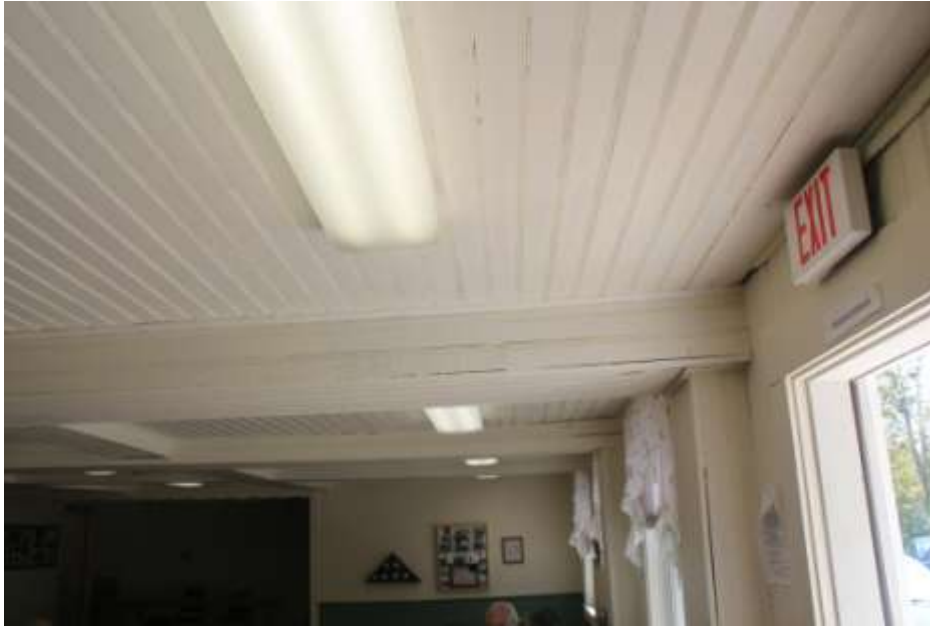
Photo 12: First floor tie beams sagging, opening joints in beadboard.
