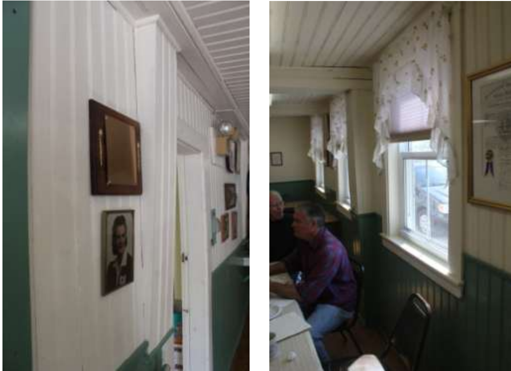
Photo 10 and Photo 11 Tapered gunstock posts in banquet hall, encased in beadboard.
