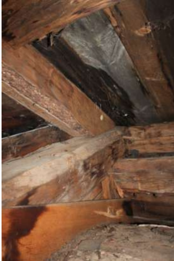
Photo 23: Tie beam, rafter and plate connection
