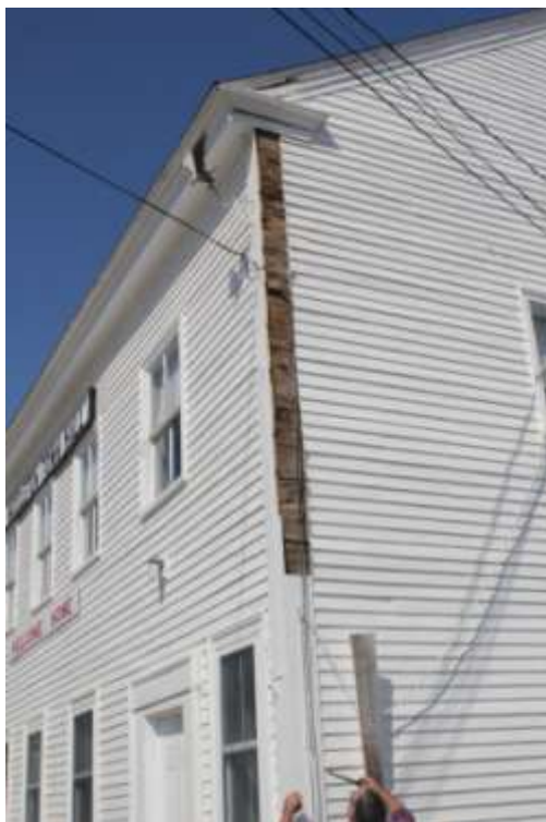
Photo 4: Corner board removed (roughly) by phone company
