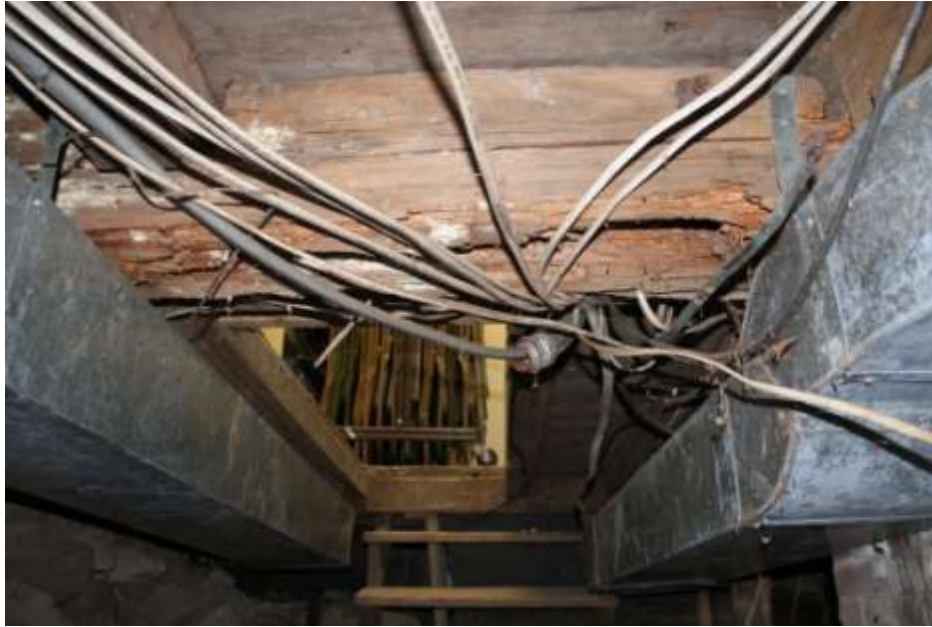
Photo 6: Rotten sill, Bent Six
