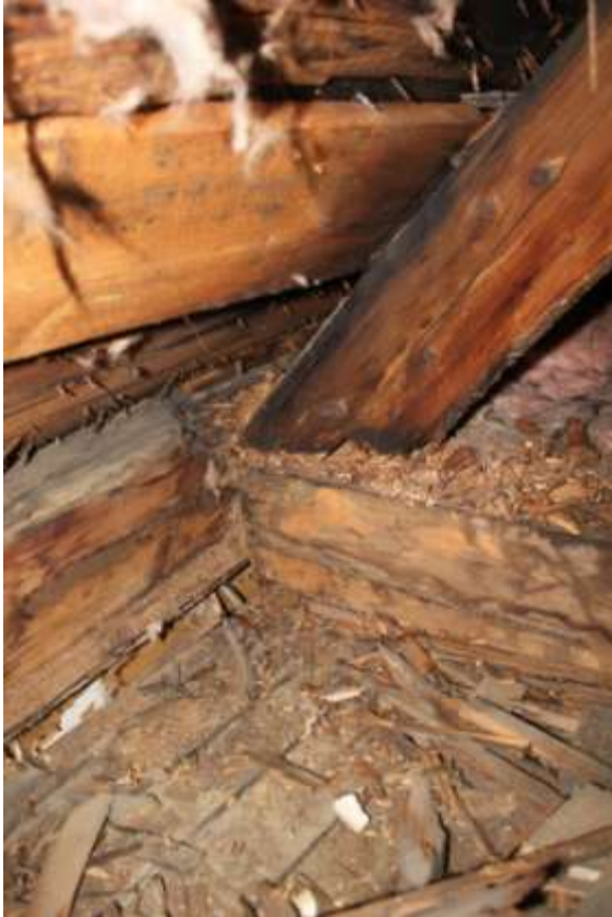
Photo 33: Tie beam 3, end rotten and severed from west schoolhouse plate
