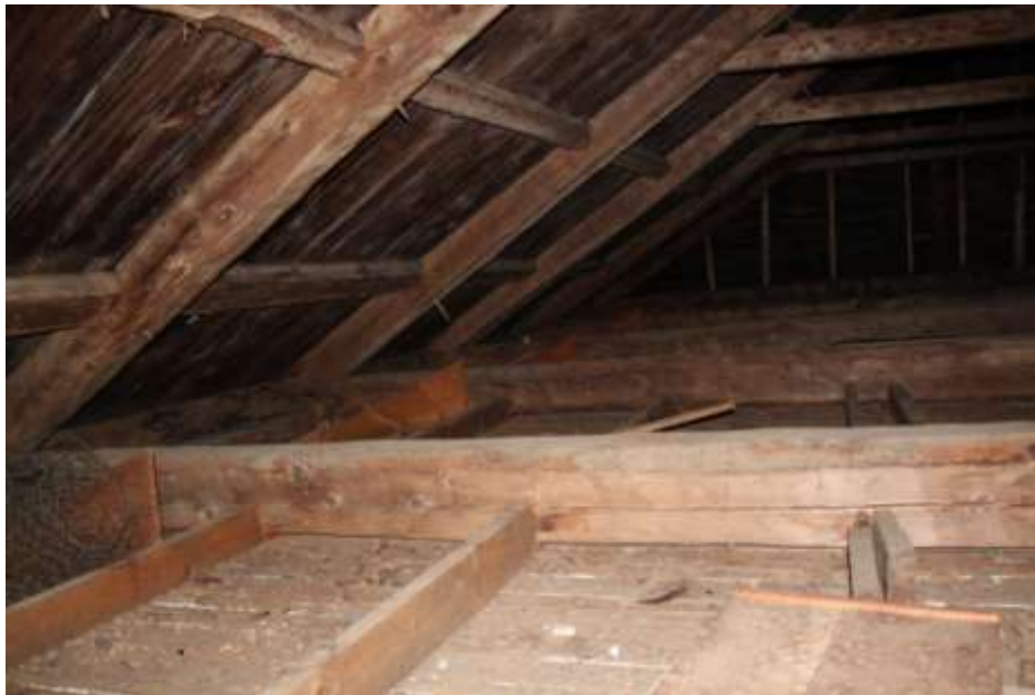
Photo 22: Oversized tie beam, 10" x 12"
