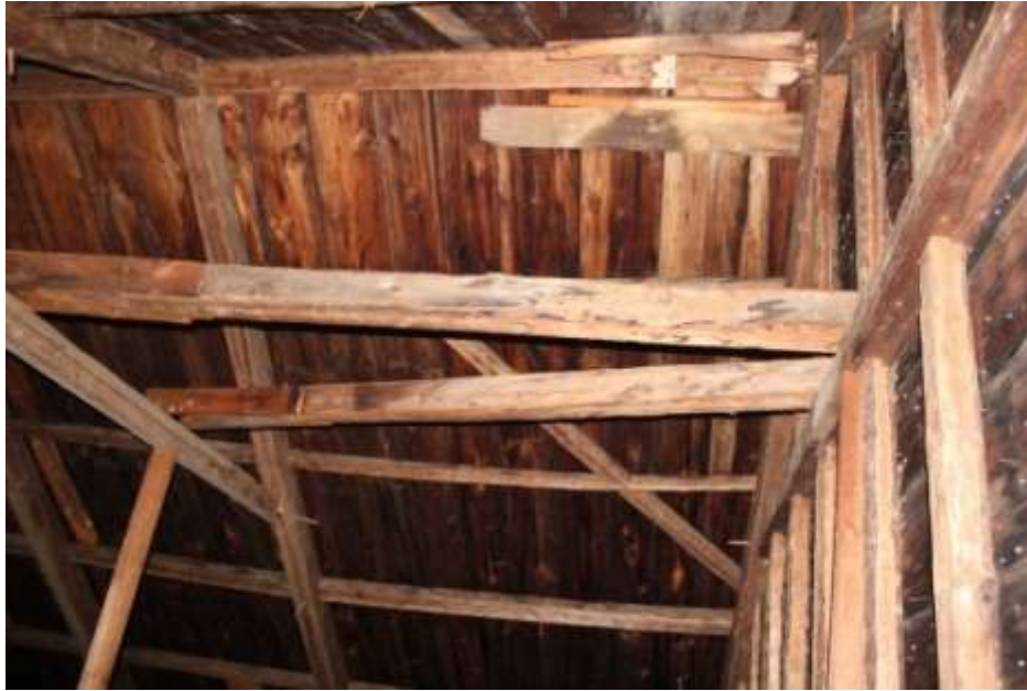
Photo 21: Wind brace in south roof pitch, adjacent Bent 6
