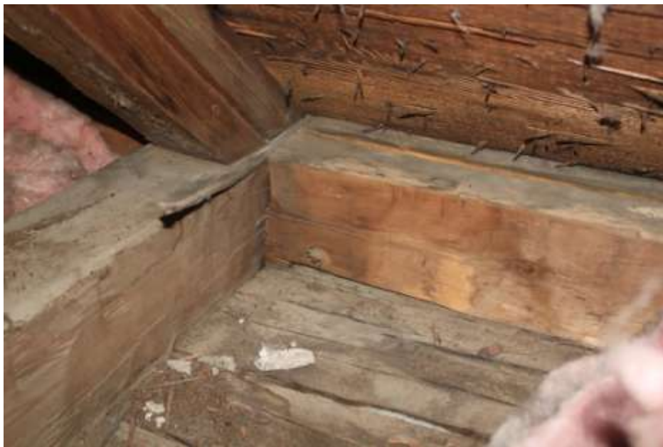
Photo 32: West schoolhouse plate, with pin at mid span
