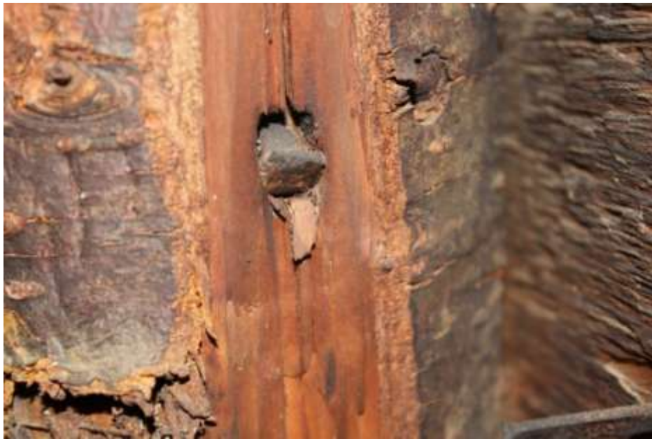
Photo 35: Early cut nail in gable end stud
