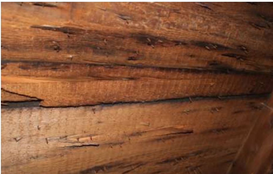
Photo 34: Schoolhouse roof sheathing, upright sawn
