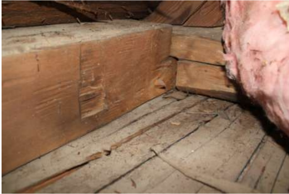
Photo 31: East schoolhouse plate, with pin at midspan
