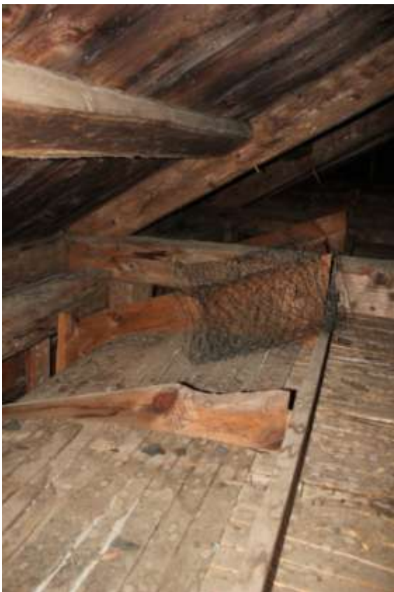
Photo 24: Coped ceiling joists, or "ribs," which create the coved meetinghouse ceiling
