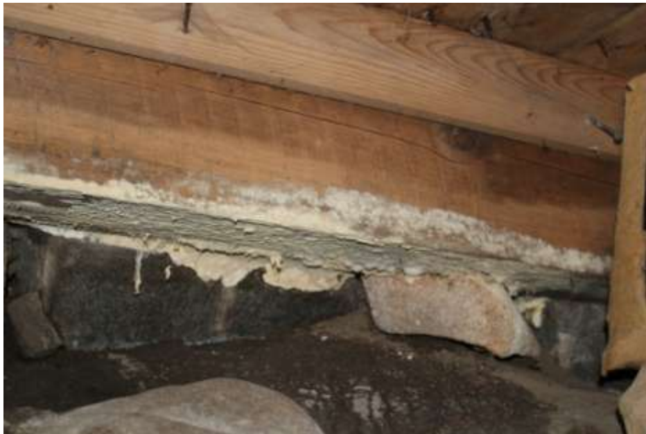
Photo 5: White mold on sill
