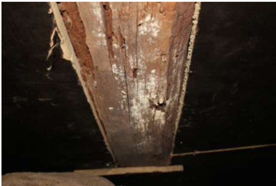
Photo 7: White mold and rot on carrying timber
