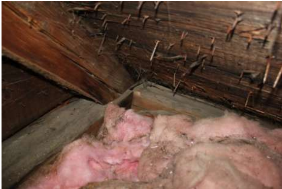
Photo 28: Schoolhouse tie beam-plate-rafter connection
