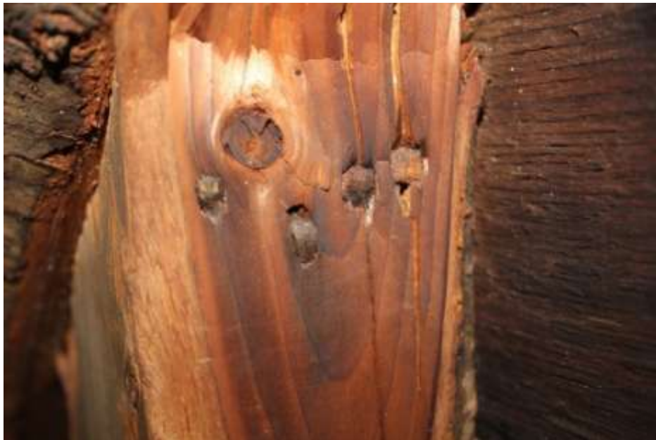
Photo 36: Wrought and cut nails in gable end stud
