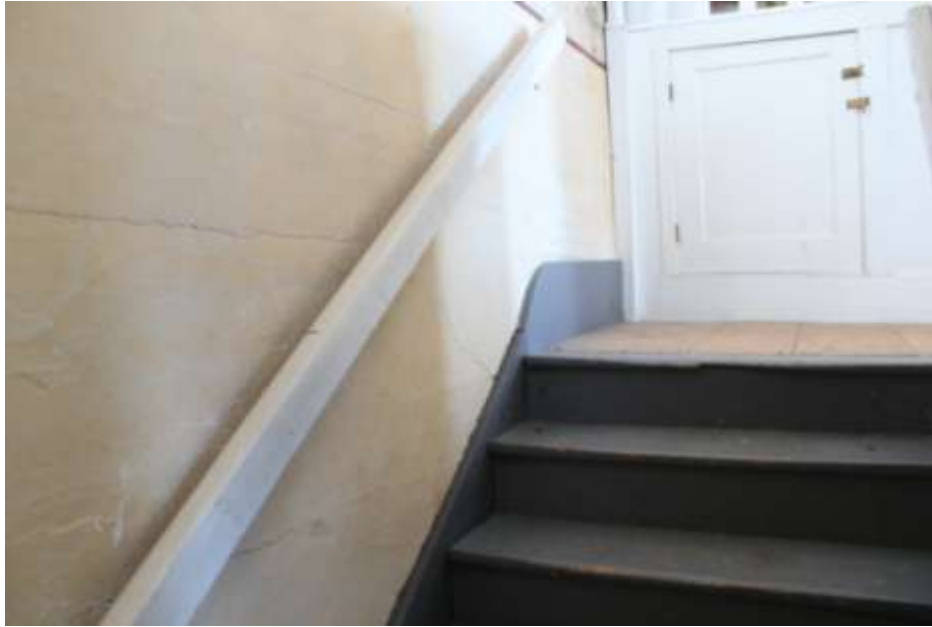
Photo 15: Existing meetinghouse stairs on west eave wall. Note change in pitch of baseboard from stairs to second floor.
