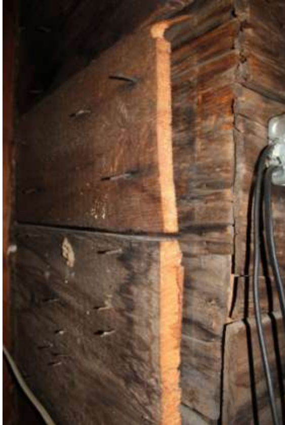
Photo 37: Gap between schoolhouse sheathing and northwest corner of the meetinghouse
