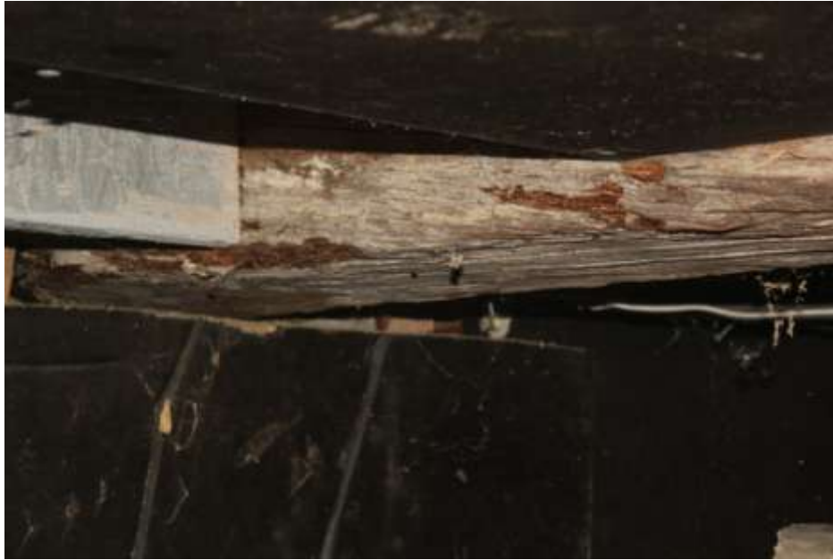
Photo 8: White mold and rot on carrying timber
